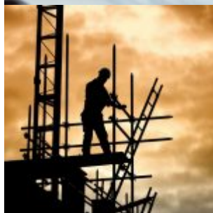
silhouette of construction worker on scaffold
