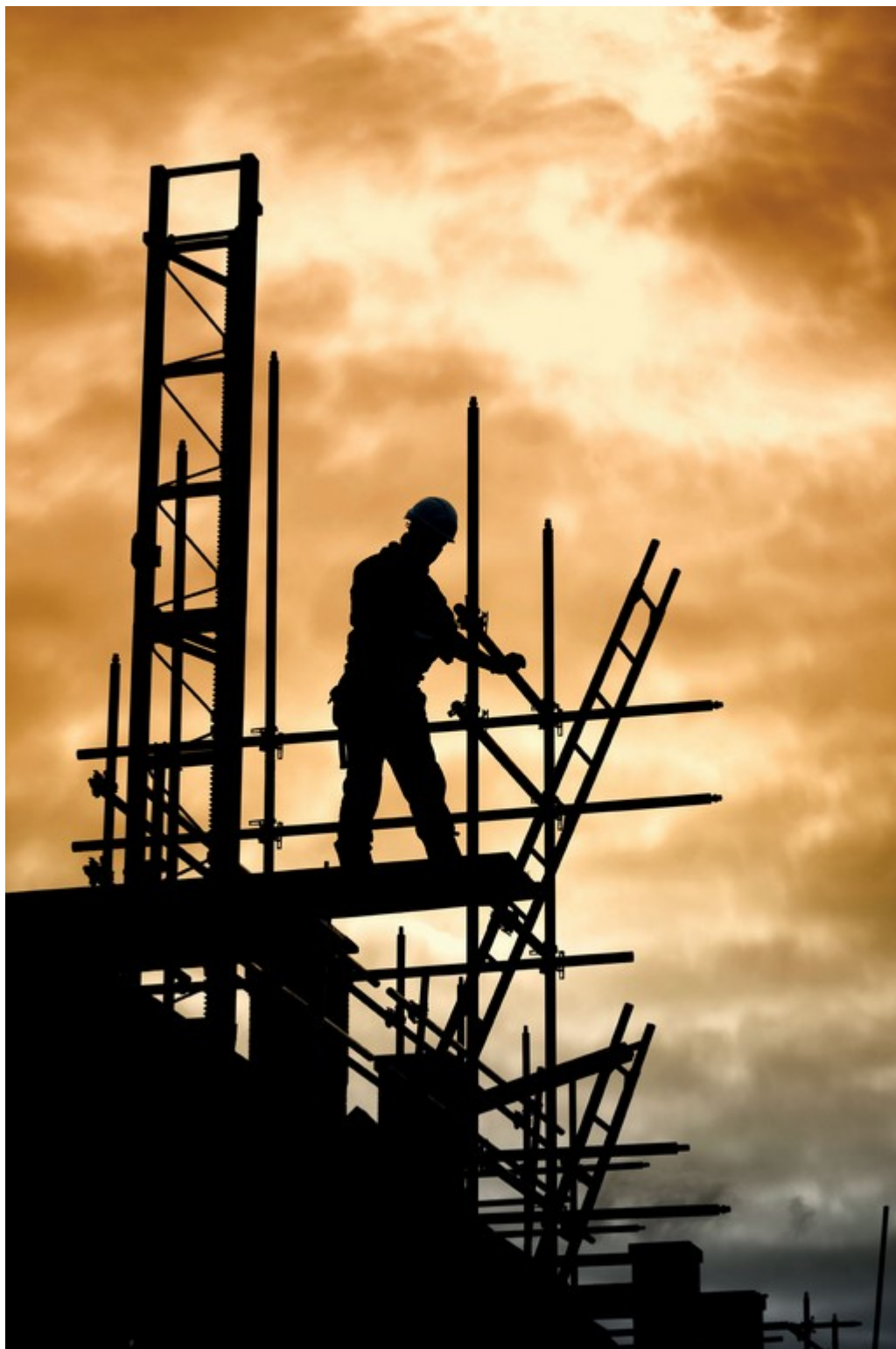
Caption: silhouette of construction worker on scaffold
